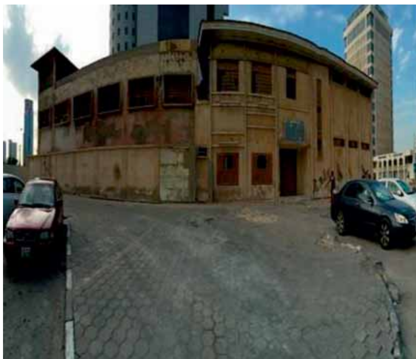
Back view of Aisha School
