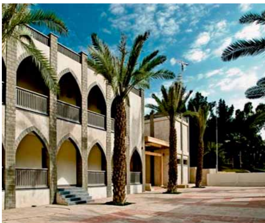
Amricani Hospital Internal courtyard
