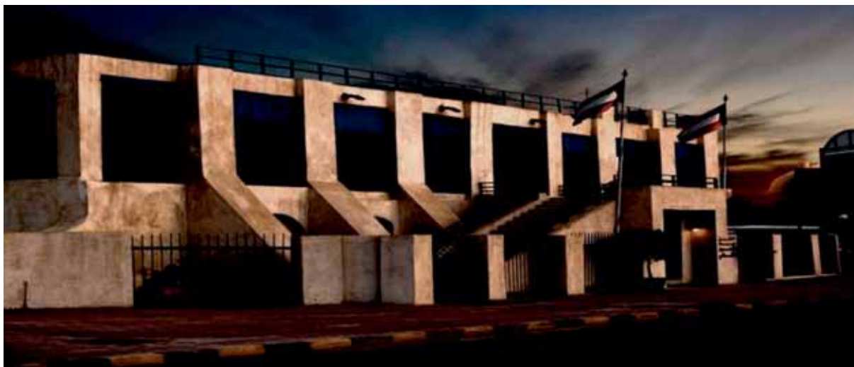
The Dickson House- General view
