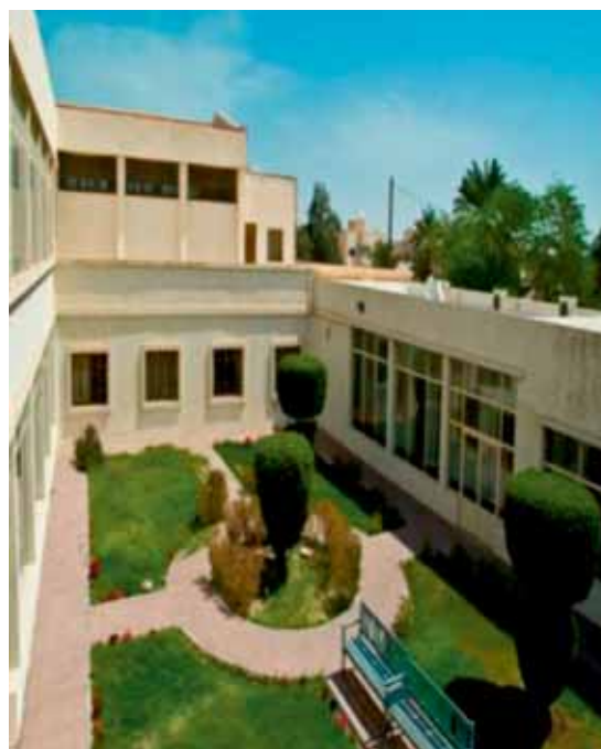
Internal View of Kathma Center
